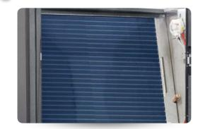
All models in the **TREF Dual Cooling** range feature standard heat exchange coils with hydrophilic coating. This special coating - together with an adequate adjustment of air through-flow speeds - helps condensate collection during the dehumidification process, avoiding dripping on the inside and outside of the unit.
