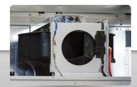
EC fans (standard for the entire range) cause the airflow to vary to match heat load requirements. This translates into a more efficient ventilation energy use and, as a result, a lower PUE for the system.
